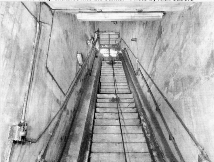
The stairs up to the emergency exit from the upper floor. Note the rails on either side of the steps - Photo by Nick Catford
